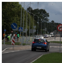
Construction of the transit city of Jūrmala P128 (Talsi highway / Kolkas street)
